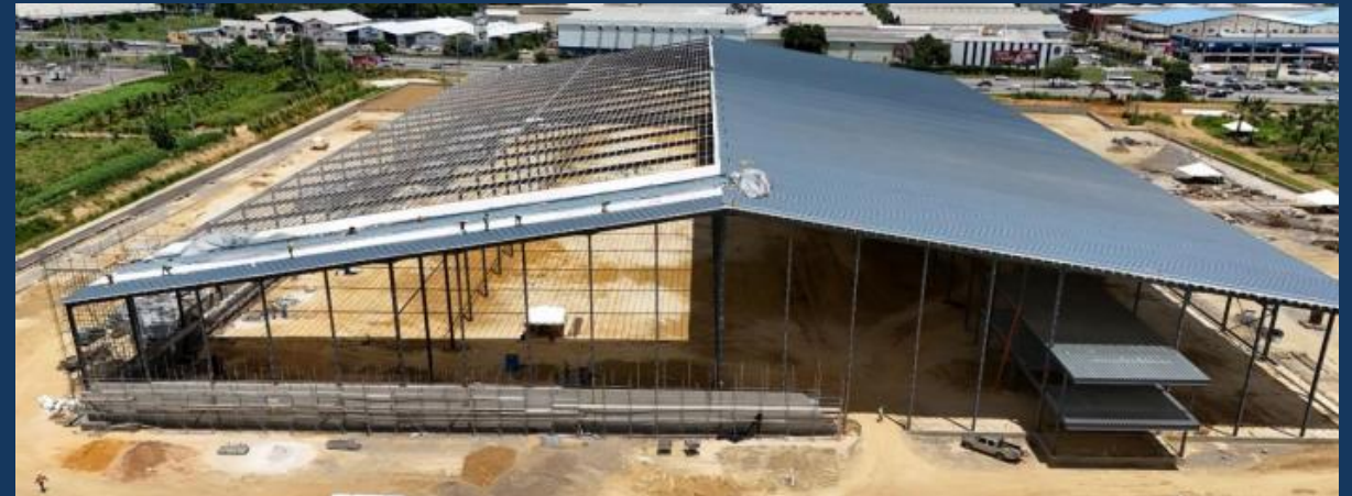
MD Trinidad – Orange Grove Warehouse
